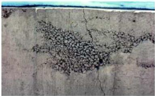
Gambar 2. 2 Honeycomb/ Cavity/ deadsound
